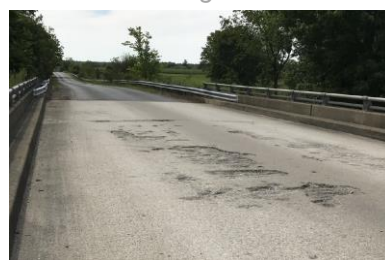
Bridge Deck Deterioration
