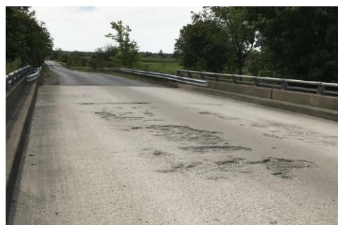
Bridge Deck Deterioration
