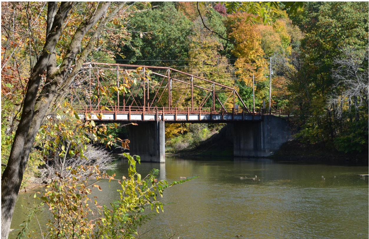
Truss bridge carrying Sixth Street / High Street over the Shenango River in Sharpsville
