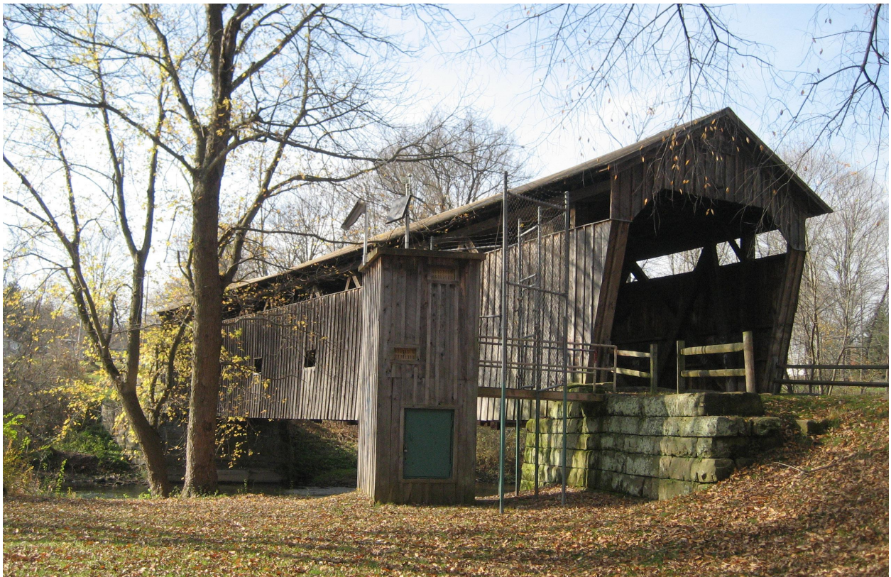
Kidds Mill Road Historic Covered Bridge
