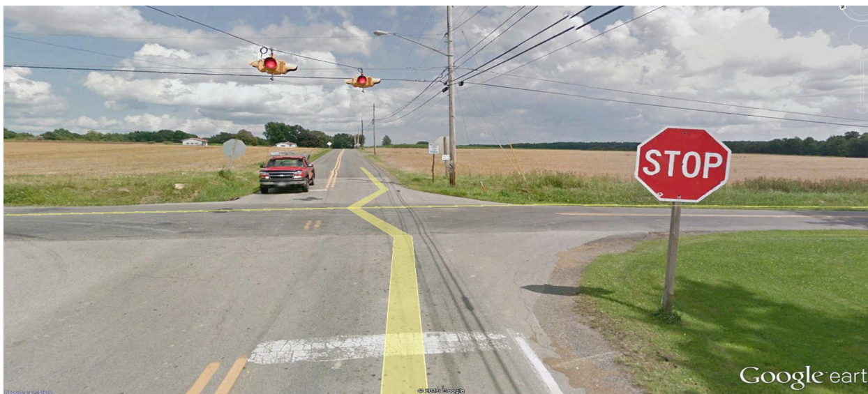
Clockwise from top left: QH #18, SR 318 - Add Curve Warning Speed Reduction Signs Curves; QH #2, Columbia Avenue Extension & Hamburg Road - Affix Stop Sign to Post Rather than Building; QH #7 - Lamor Road & Neshannock Road - Add "Cross Traffic Does Not Stop" Sign Source: Google Earth
