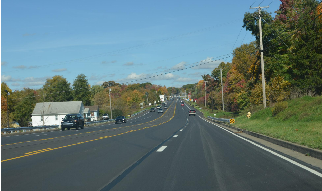
Freshly repaved section of northbound US 18 near the I-80 Interchange
