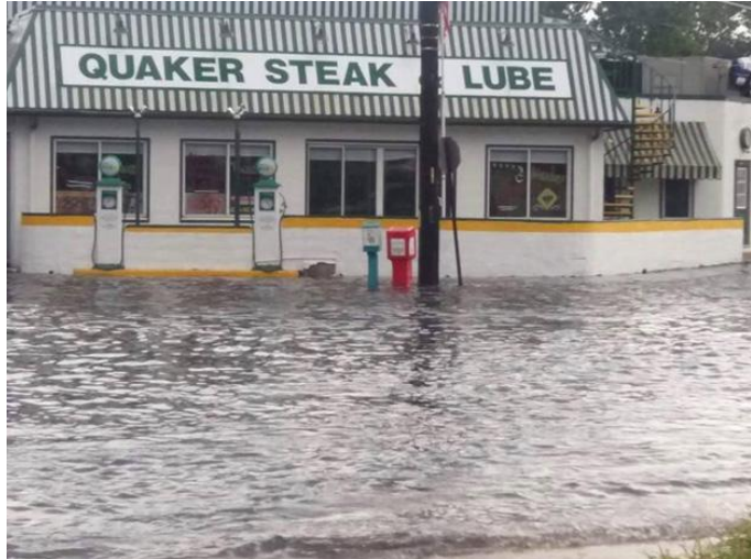
Flooding due to Storms at The Original Quaker Steak & Lube in Sharon, PA in August 2016 Source: WFMJ
