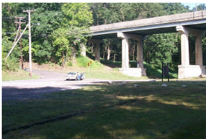
The development of trailhead facilities and connections to the downtown and neighborhoods of West Middlesex and PA 318 should be explored as part of a Shenango River Trail Feasibility Study.
