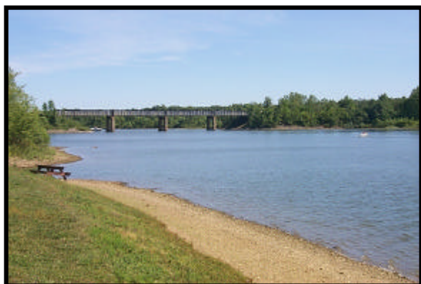
Figure 29. U.S. Army Corps of Engineers' Dam Overlook.
