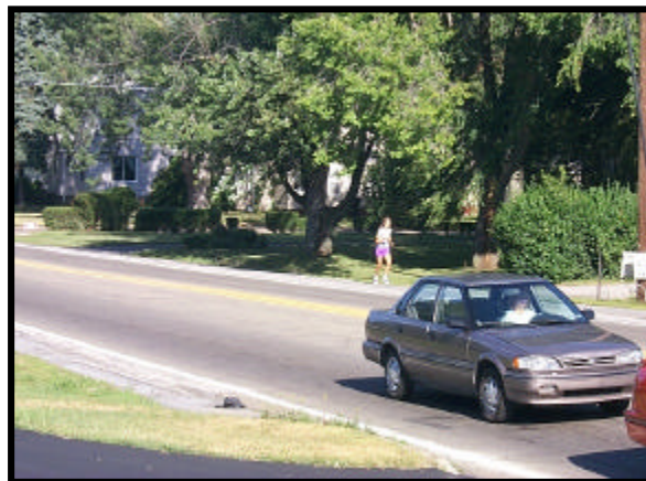
Figure 10. No sidewalks along Highland Road between the Municipal Boundary and North Buhl Farm Road (northwestward view).
