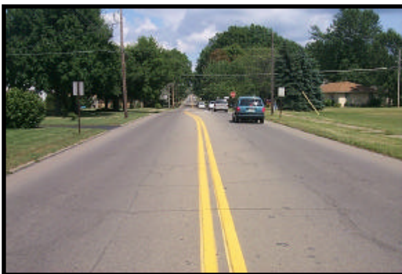
Figure 5. Highland Road between Jefferson Avenue and the Municipal Boundary (eastward view).
