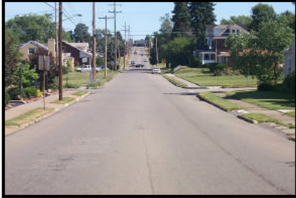
Figure 30. Indiana Avenue (northward view).
