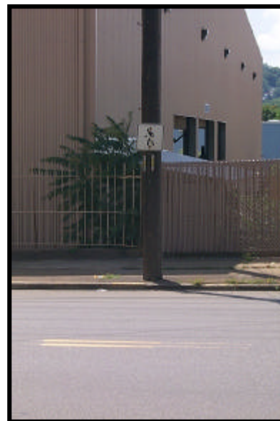
Figure 11. “NO PEDESTRIAN CROSSING SIGNS” should be removed where possible.
