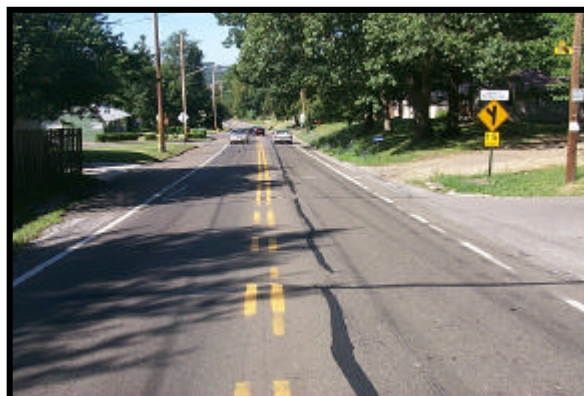
Figure 34. Segment of Mercer Avenue to have curb and sidewalk installed (southwestward view).
