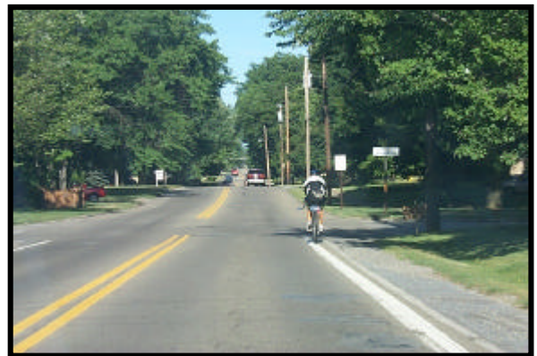
Figure 6. Highland Road between N. Buhl Farm Drive and the Municipal Boundary (westward view).
