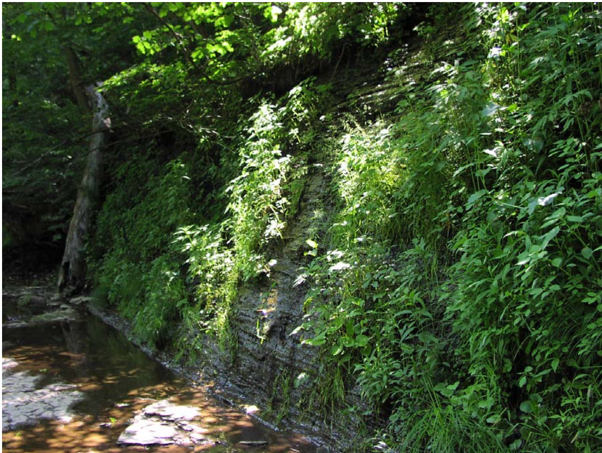
Figure 14. Seepage along Deer Creek
