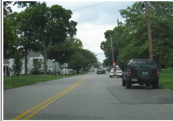
Photo # / Description: Segment 6-7 (NB) south of courthouse area
