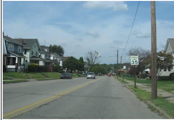
Photo # / Description: Segment 3-4 (NB) w/ on-street parking
