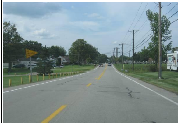
Photo # / Description: Segment 1-2 (NB) near cemeteries / Likens Ln
