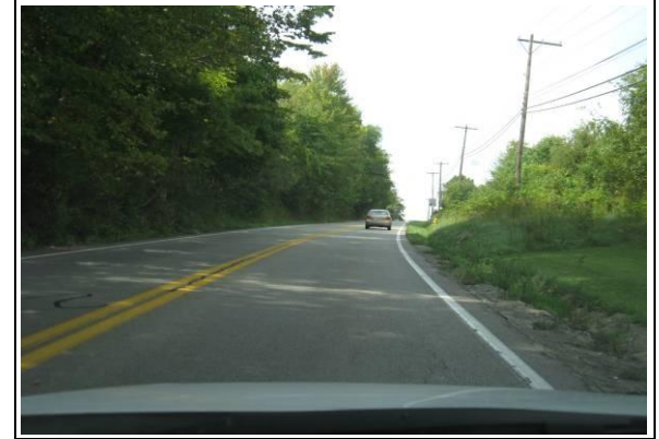
Photo # / Description: Segment 1-2 (NB) view north on 10% upgrade
