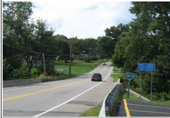
Photo # / Description: Segment 1-2 (NB) view north of PA 18
