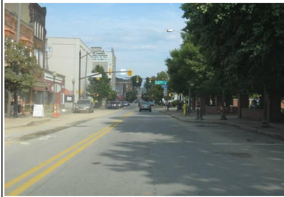
Photo # / Description: EB approach to #2 (Water Ave)
