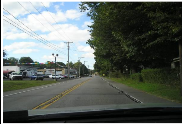
Photo # / Description: NB approach segment 21-22
