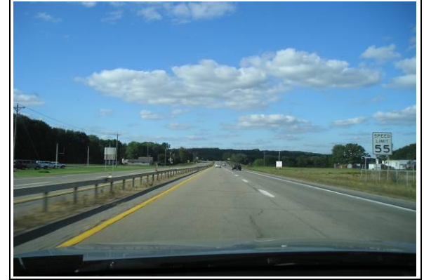
Photo # / Description: NB approach segment 16-17
