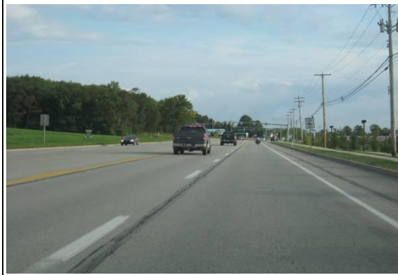
Photo # / Description: Segment 13-12 (SB) near Wal-Mart
