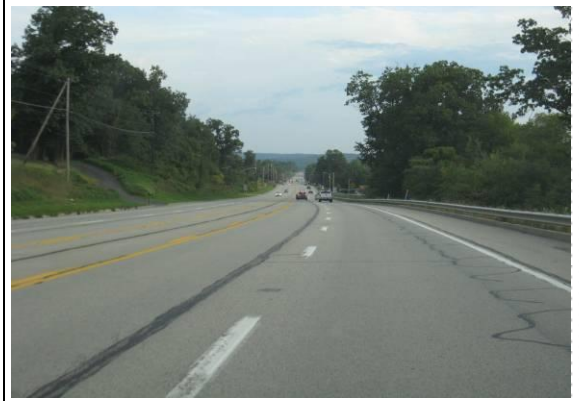
Photo # / Description: Segment 6-5 (SB) wide five-lane section
